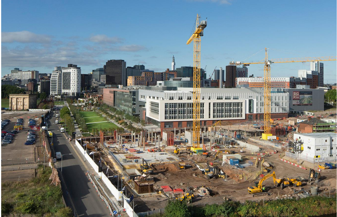
Figure 4.1 Birmingham City University Development Construction Site
