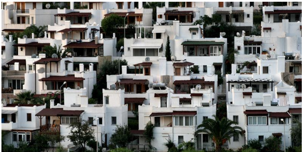
Figure 2.8 Traditional settlement pattern in the city of Bodrum where the climate is hot and humid
