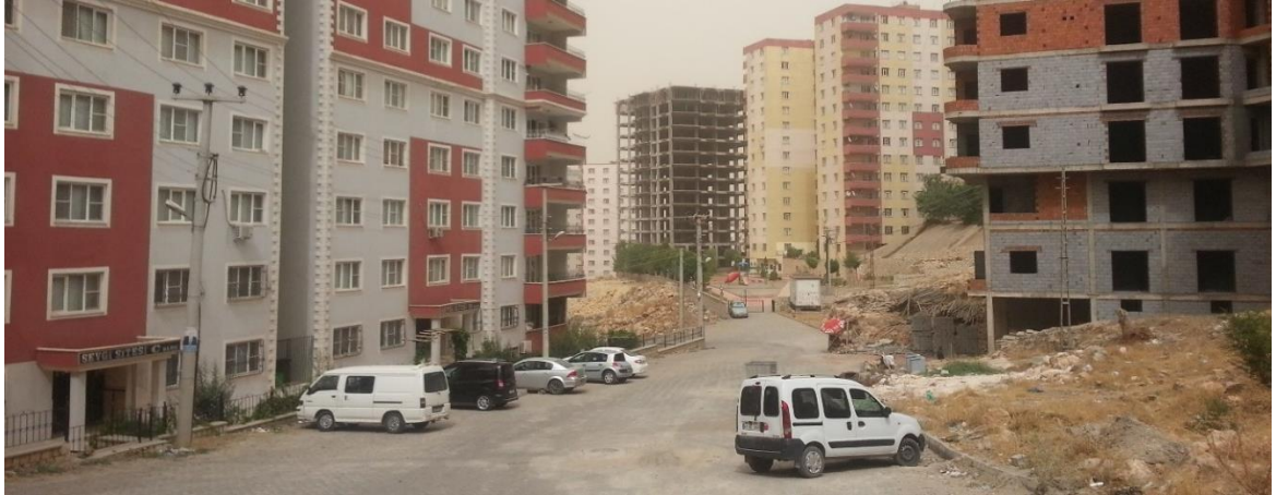
Figure 7.22 A typical neighbourhood developed by sub-contractors
