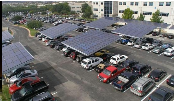
Figure 3.3 A solar shaded parking structures, at Dell's headquarters in Round Rock, Texas
