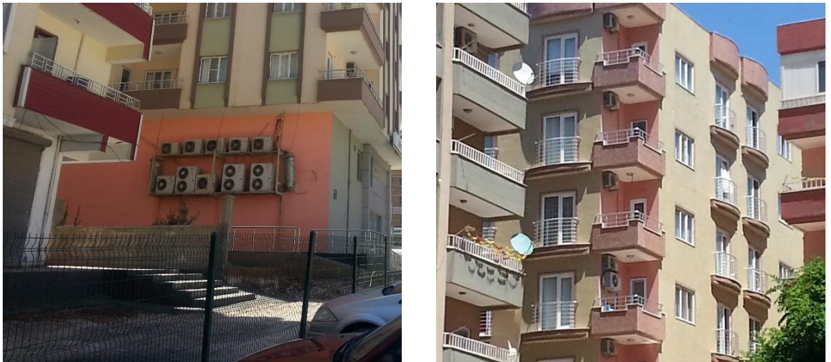
Figure 7.8 Sample facades covered with engines of air-conditioners
