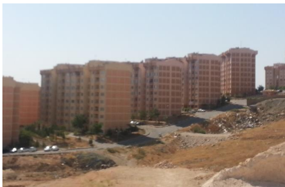
Figure 5.19 Views of TOKI housing development site
