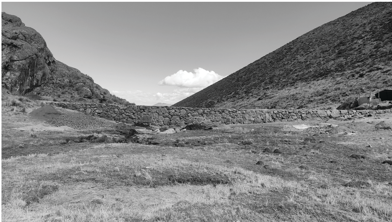
Figure 15.6 Fully restored Ricococha Alta dam. Past Water Futures Project.
