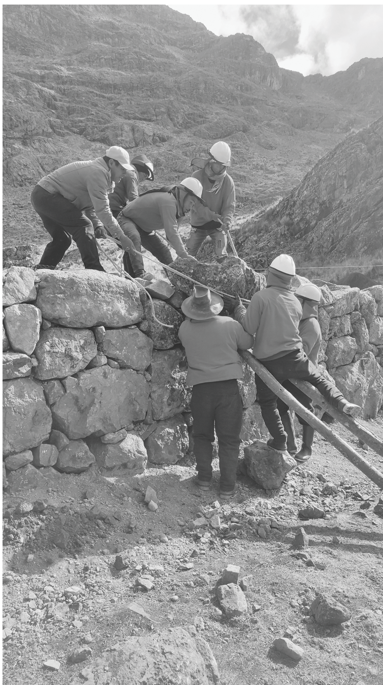
Figure 15.5 Restoring fallen rocks manually onto the dam crest, Ricococha Alta. Past Water Futures Project.
