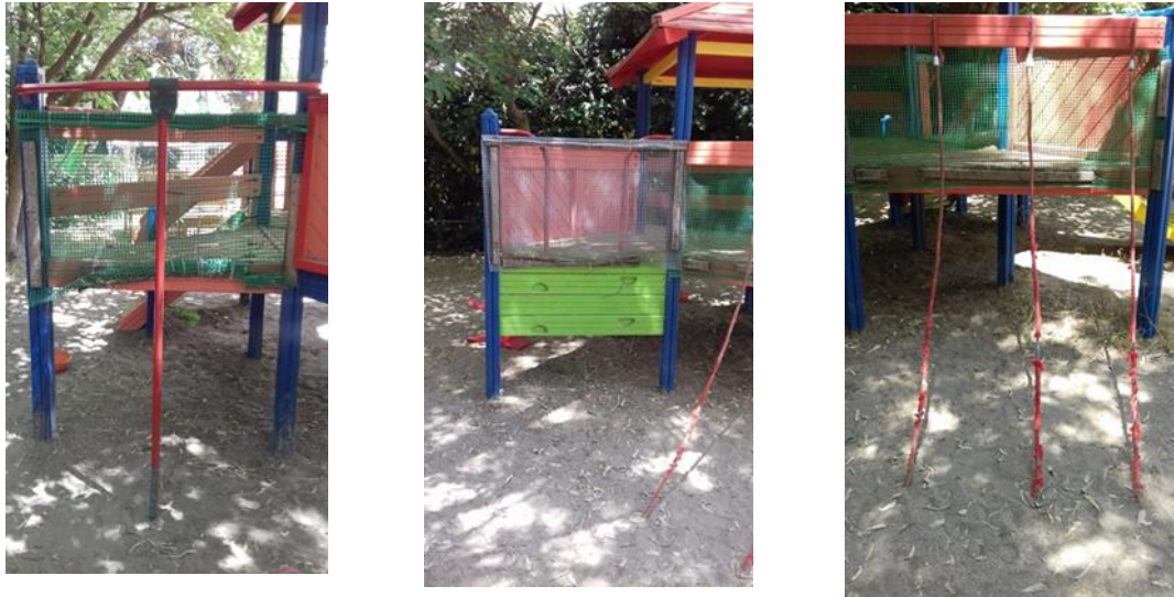
Figure 5.12: Covered sides of elevated construction.
