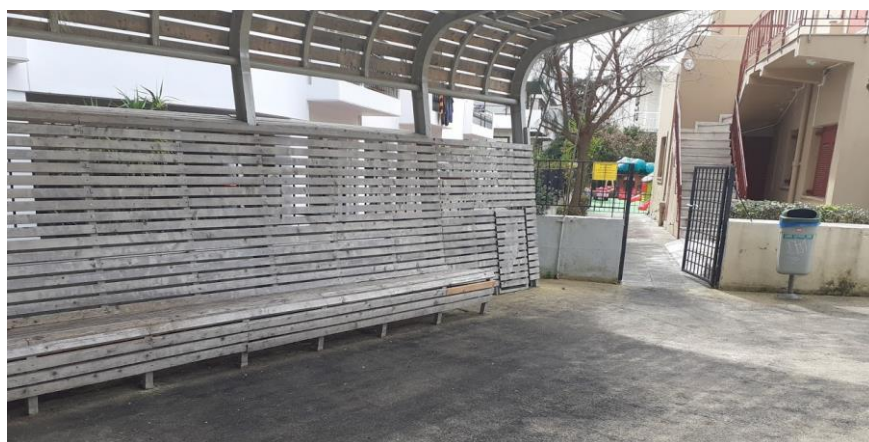
Figure 7.10: View of the small play area from the main playground's shaded area with benches.
