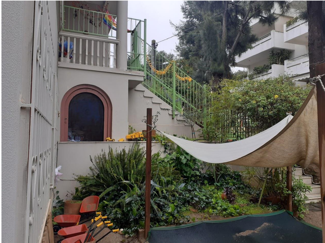
Figure 6.5: Staircase leading to the garden from first floor
