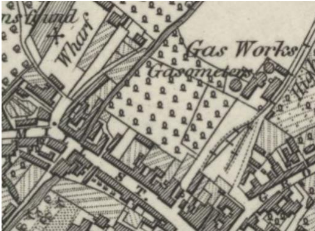
Figure 164: Location of Wantage Tramway Terminus and Canal Wharf on Mill Street, Wantage. 45
