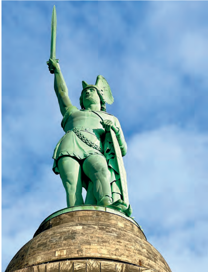
Ernst von Bandel, Hermann Monument ( Hermannsdenkmal ) (1838–1875), copper plates riveted together and supported by an iron frame, Height of the monument, 53.44 m, Teutoburger Wald, Detmold. [Wikimedia Commons]
