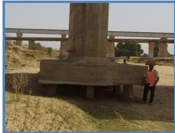
Figure 23. Exposed pile caps and piles
