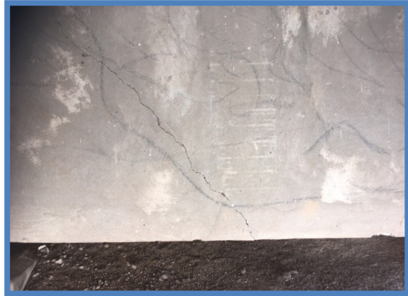
Figure 18. 3mm wide crack on approach beam
