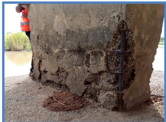
Figure 5. Exposed rebar with section loss
