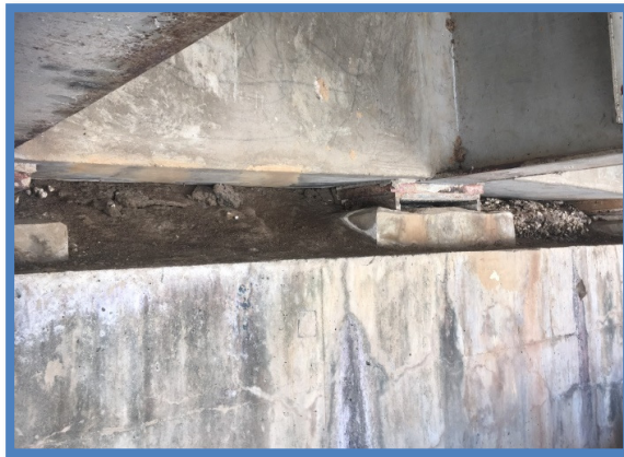
Figure 17. Soil loss from roadway approach.
