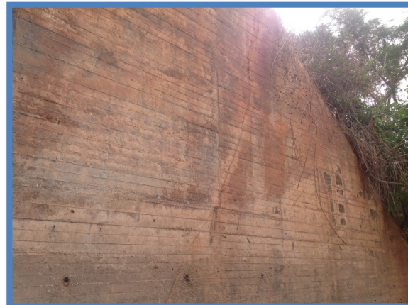
Figure 8. Pronounced crack on wingwall.
