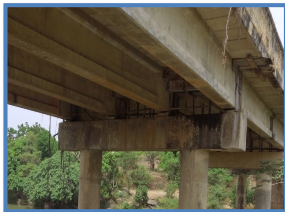
Figure 15. Formwork observed under deck.
