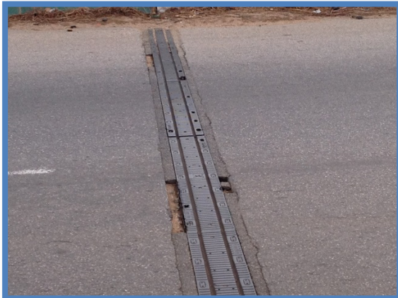
Figure 3a. Deteriorating expansion joint
