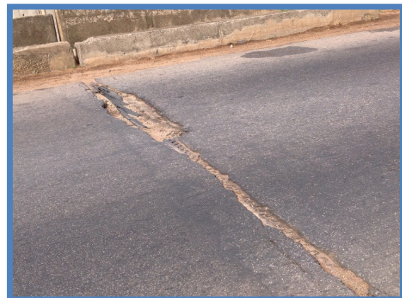
Figure 3b. Deteriorating expansion joint.
