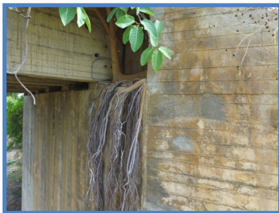
Figure 7. Tree growing on abutment seat.
