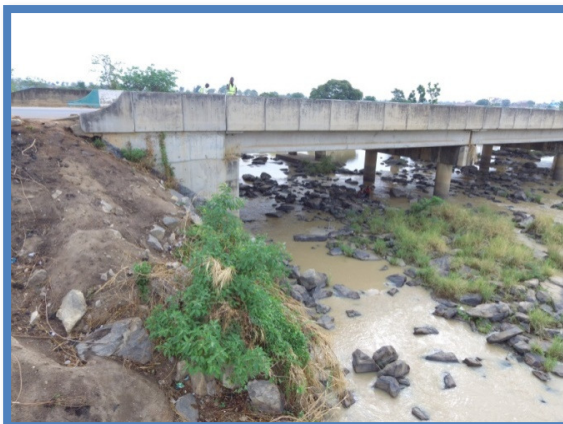
Figure 4. Dislodged stone pitching Source: Field Survey 2019
