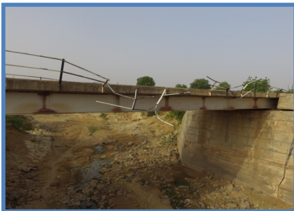
Figure 28. Poor attempt to arrest backfill loss.
