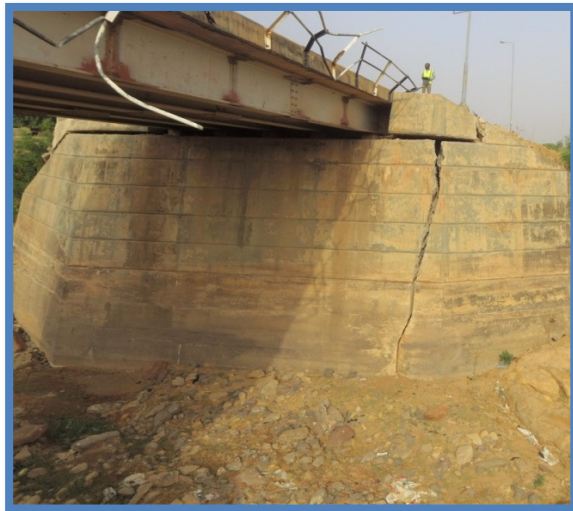
Figure 26. Major cracks on abutment.
