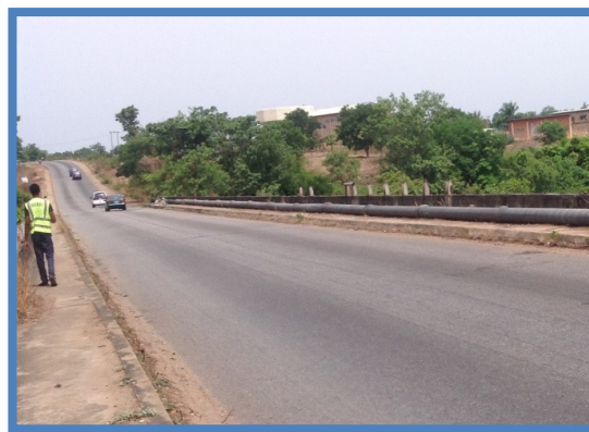
Figure 13. Missing railings due to vandalism
