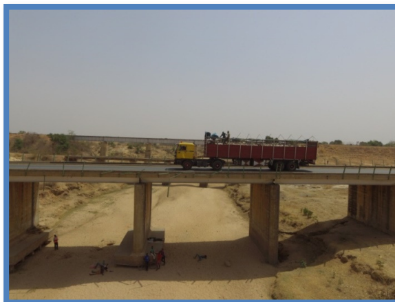
Figure 22. Noticeable absence of railings.
