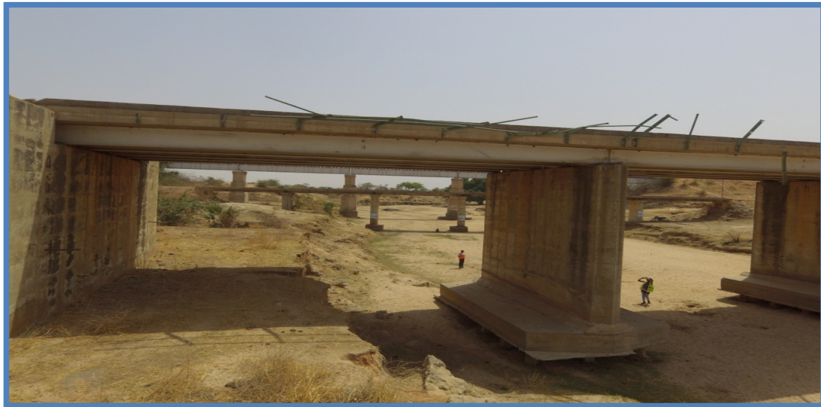
Figure 24. Major loss of channel bed to erosion and scouring. Source: Field Survey 2019
