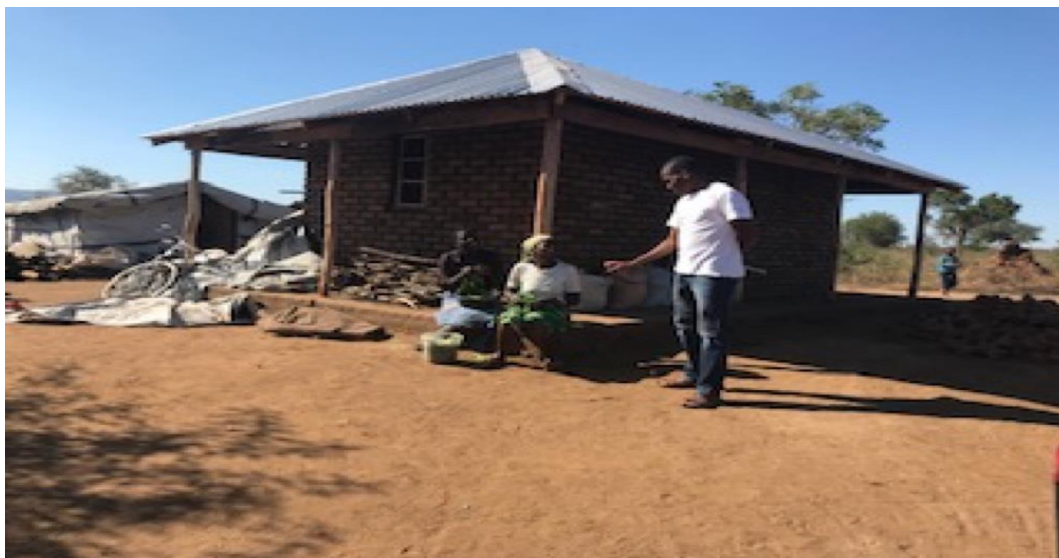
Figure 13: A one bedroomed raised foundation house handed over to some of the resettlers by CADECOM in Mwalija Village resettlement site. (Photo by author)
