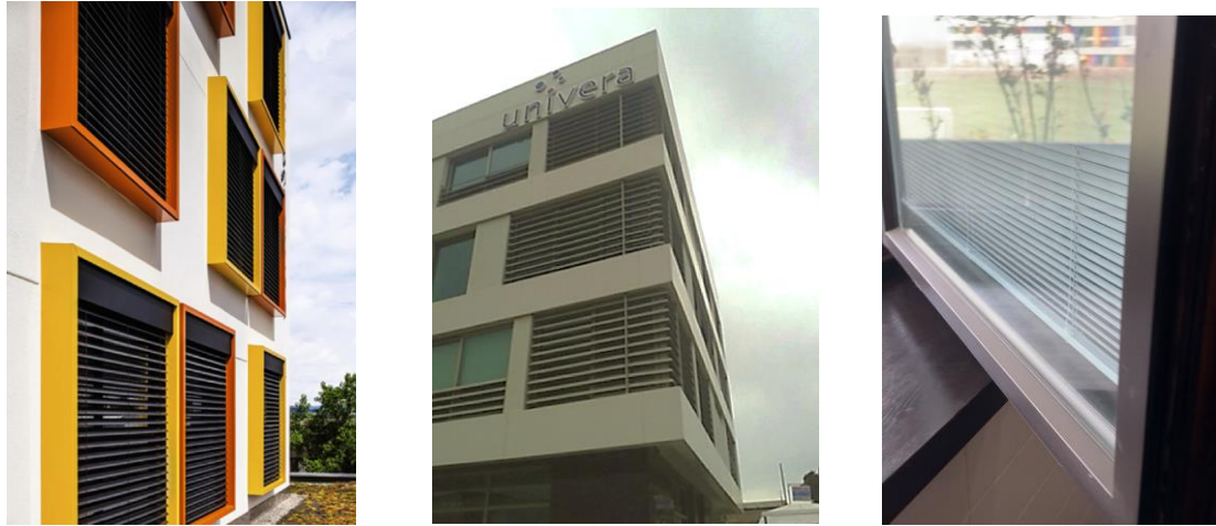
a) Curved blinds in roller shade [48]; b) Horizontal louvers [49]; c) a window with built-in venetian blinds (picture: the author)
