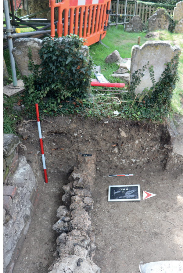
Fig 34. Foundation of south nave wall. Photograph: authors.
